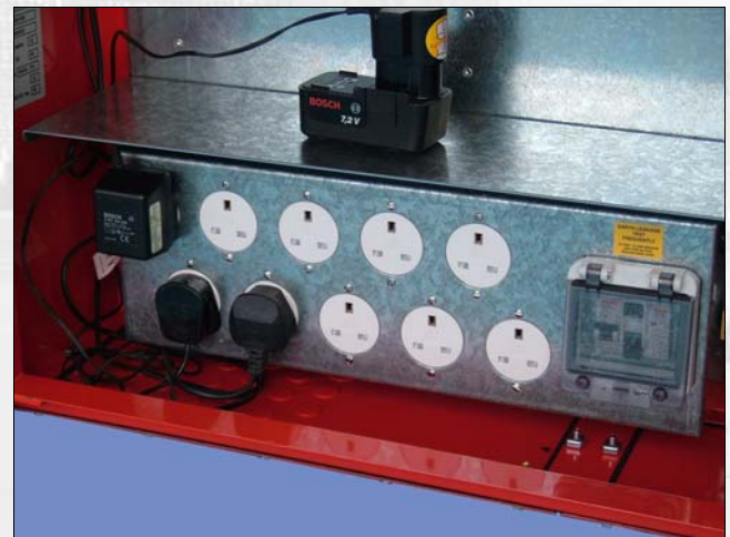
Close up showing MCB, RCD and Sockets
