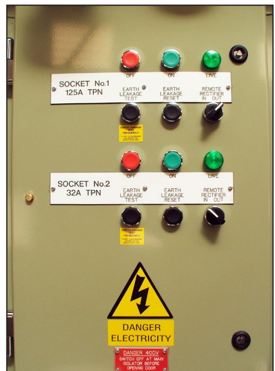
External controls for routine ON, OFF, TEST, RESET and PCP selection operations
