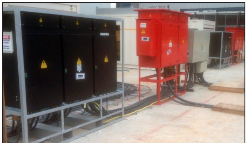
2000A Mains Distribution Assemblies supplied from generators via Automatic Mains Failure Assemblies
