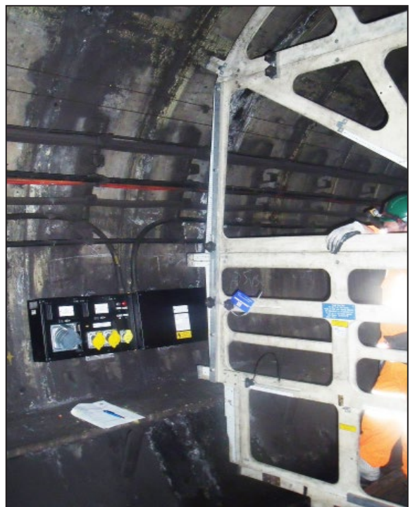
Part A7042930 - Tunnel Power Transformer, Horizontal Orientation, with additional 400V socket
