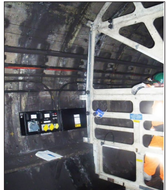
Horizontal TPT with LUL gauge alongside to ensure safe clearance distances.
