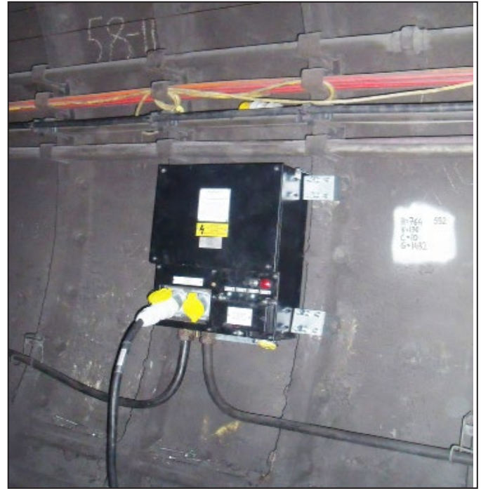
Vertical orientation Tunnel Power Transformer with bottom cable entry / exit.
