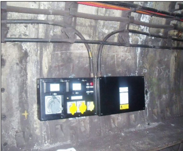
Horizontal orientation with the addition of a 32A, 400V, 3P+N+E, metal clad interlocked socket with the grey socket cover instead of the usual red. Top cable entry / exit.
