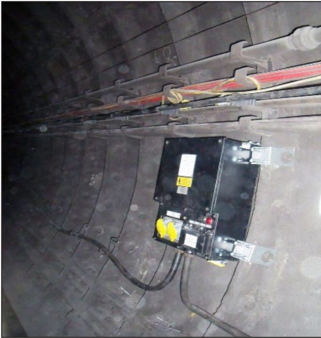
Vertical orientation Tunnel Power Transformer with bottom cable entry / exit.
