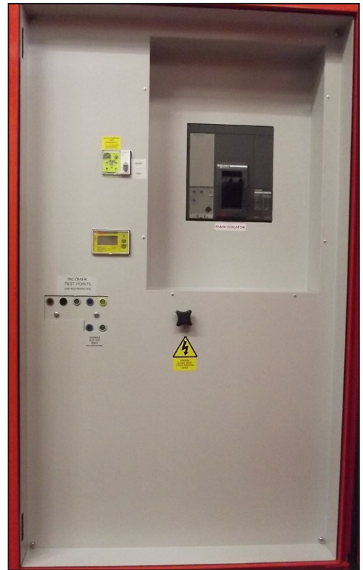
Test sockets fitted in the incoming section of a 1600A MDA
