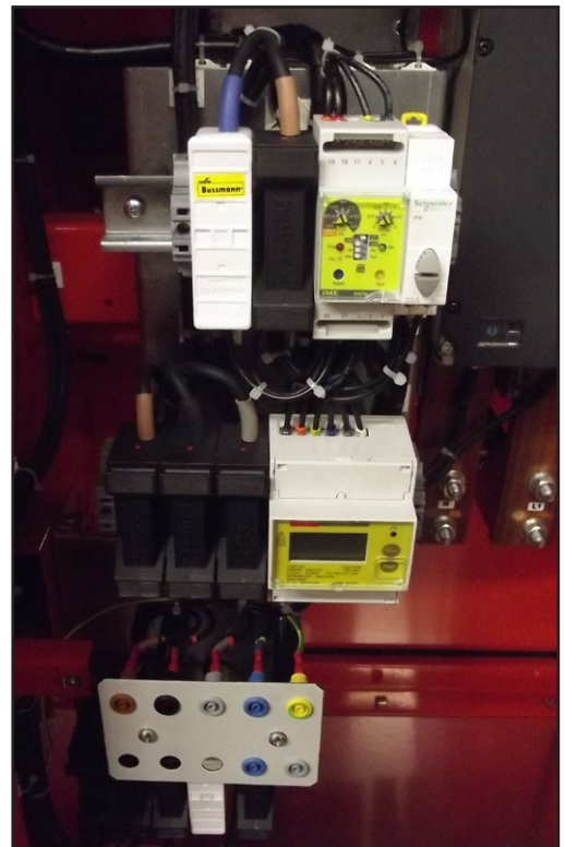
Test sockets fitted in the incoming section of a 1600A MDA
