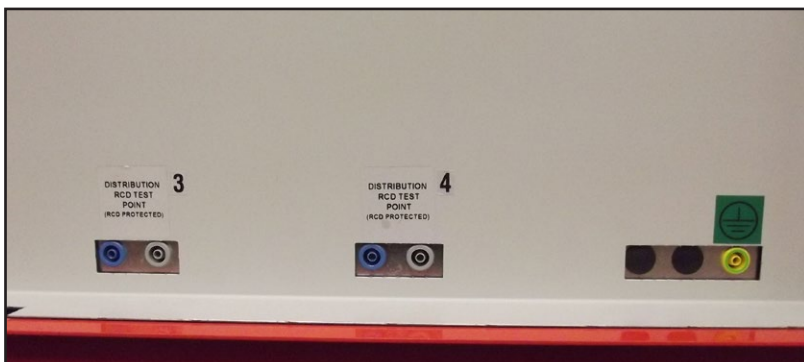
Test sockets fitted in the outgoing section of a 1600A MDA
