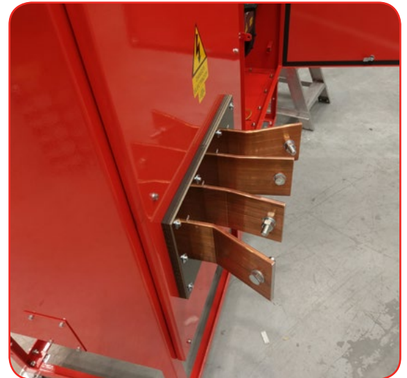
Special Incoming Termination Arrangement
