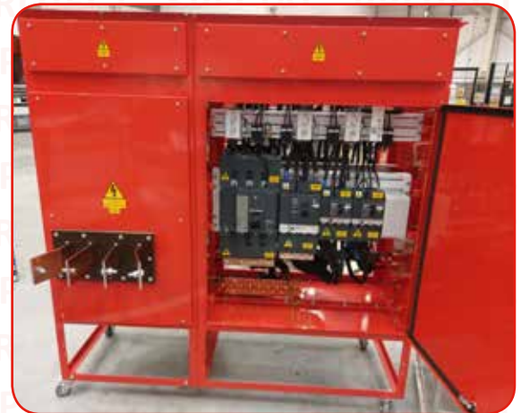
B7 1600A MDA configured for Testing
