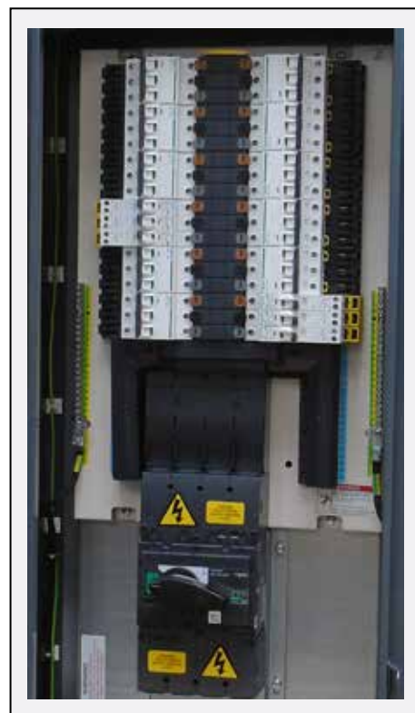
Distribution Board, 200A, 12 way, TP&N, IP66; Inset Panel Removed
