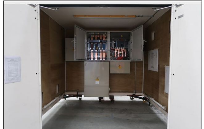
A7292794 Equipped ISIA Pillar, 3m x 3m x 2.4m fitted with an 800A SSE specification CT Chamber with main 4P switch
