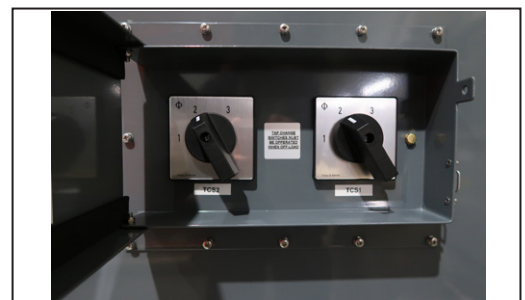
Off Load Tap Changing, Accommodating a Supply Voltage Range of 360V to 440V
