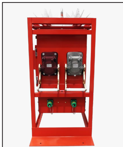
Plug-in Protective Conductor, interlocked with respective socket
