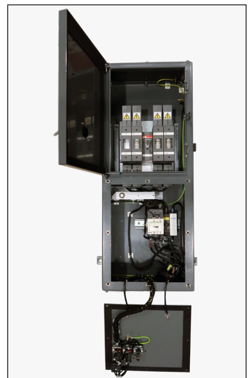
A7292575 with door open and bolt-on front cover and socket removed
