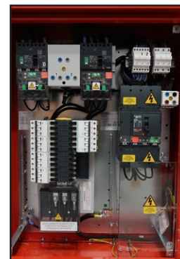
Tunnel MDA, 250A with incoming CBR and outgoing CBRs and MCBs, c/w test sockets. Part no. A7085175.
