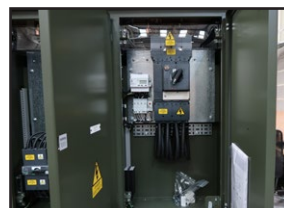
2 no. Incoming compartments each with a 630A MCCB, which are key interlocked to prevent simultaneous closure.
