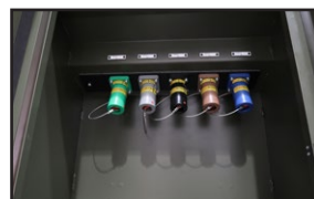
1 no. set of 800A SPCs feeding a 630A incoming MCCB
