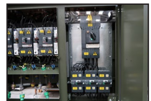
2 no. Incoming compartments each with a 630A MCCB, which are key interlocked to prevent simultaneous closure.
