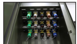
3 no. sets of 400A SPCs, each feeding a 125A incoming MCCB
