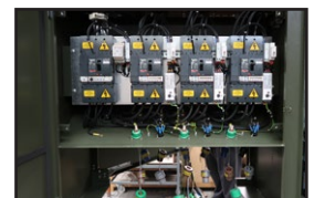
3 no. outgoing sets of SPCs & 1 no. 63A 5P socket. The SPC circuits incorporate monitored earth protection and the multipin socket is protected by MCCB with variable RCD.
