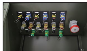
3 no. outgoing sets of SPCs & 1 no. 63A 5P socket. The SPC circuits incorporate monitored earth protection and the multipin socket is protected by MCCB with variable RCD.
